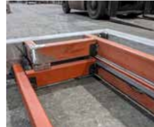
Inner edge beam return to door pocket
