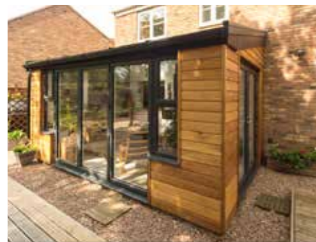
Horizontal Timber Boards
