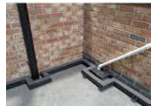
Intrusions for pipework
