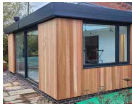
Vertical Timber Boards
